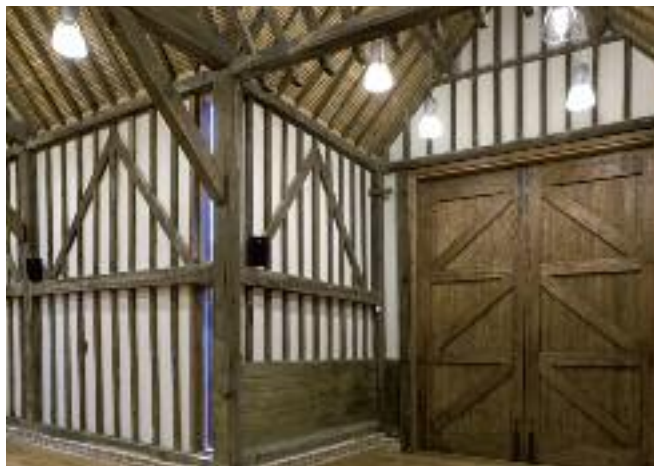
Royal Opera facility
