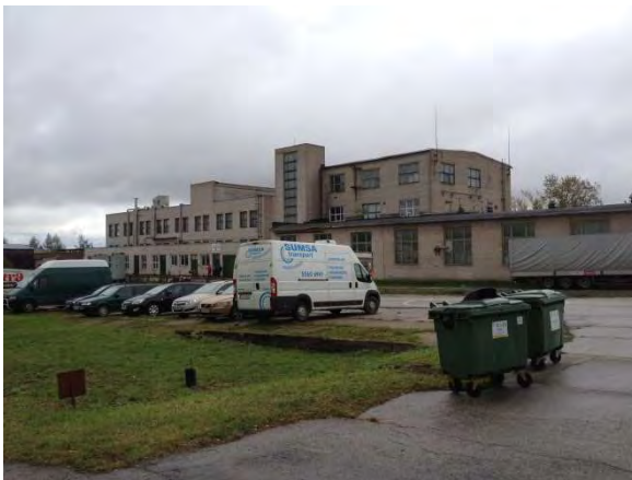
External view of the industrial building
