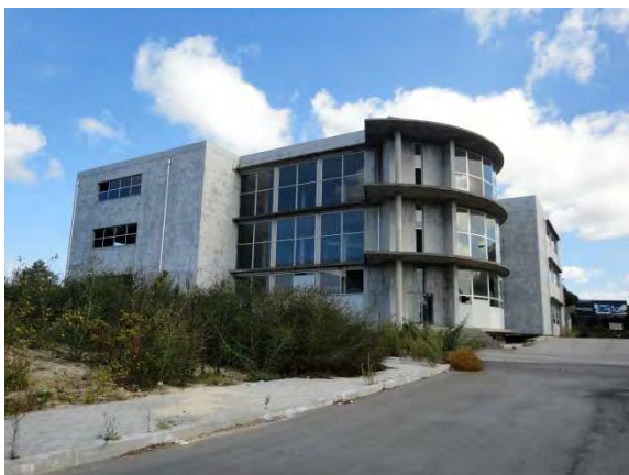
Abandoned Showroom during construction
