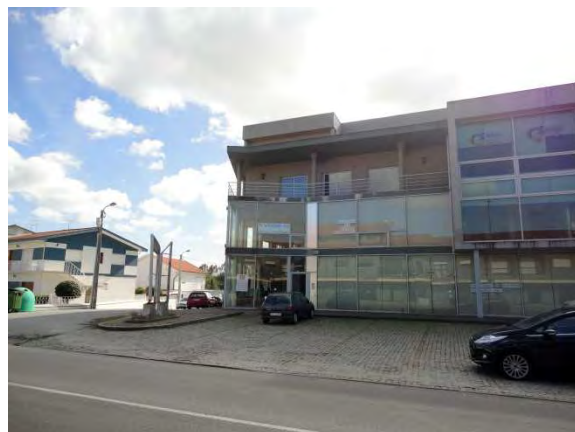
Abandoned showroom after years of use
