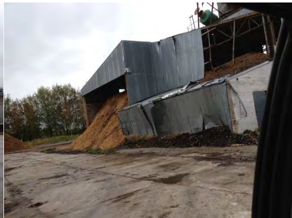
Abandoned wood storage building
